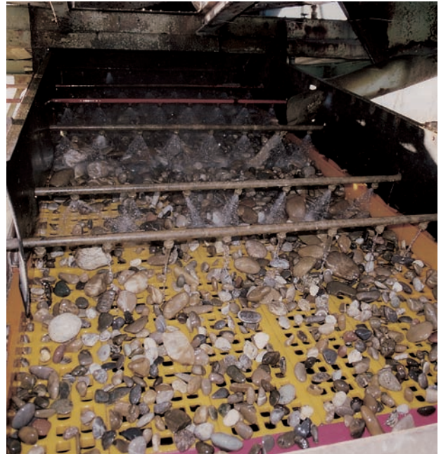
WS 85 in sand and gravel processing
